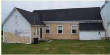
Freeport Baptist Church Repair
