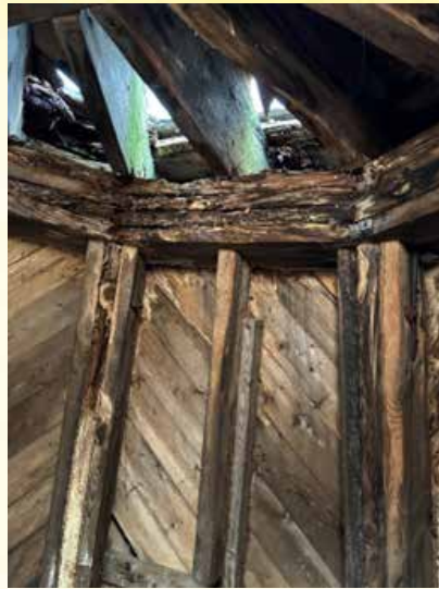
Lantern floor before repairs
